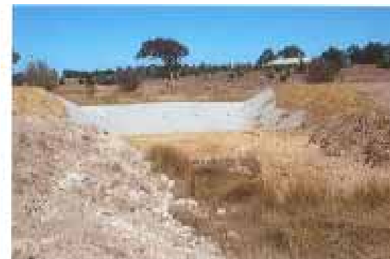
Concrete Flume installed at Harold & Marie Bensley's
